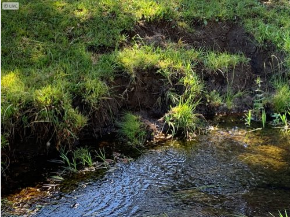
Detail of streambank chiseling above. July 29, 2020.
