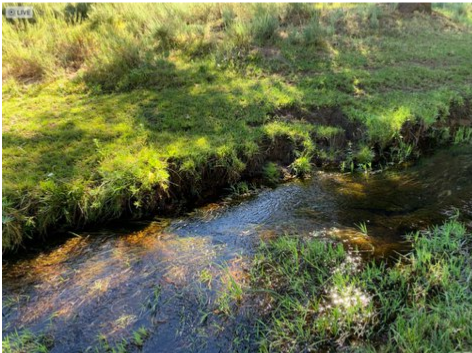
Chiseling of streambank by cattle hooves, and the beginning of a larger section of streambank collapsing into the water. July 29, 2020.
