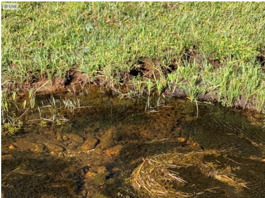
Chiseling of the streambank by cattle hoof traffic. July 29, 2020. This is how streambanks break down and deep narrow channels become wide and shallow.
