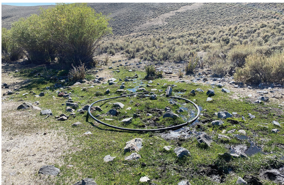
Damaged spring with broken poly pipe on the Mountain Springs BLM allotment near Mackay, Idaho.
